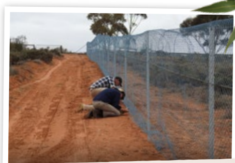
Friends building the replacement vermin proof fence in 2018. The gap above the Spencer Gulf boundary still needs to be closed to exclude kangaroos, emus, goats, rabbits, foxes and feral cats to protect the vegetation, bird life and small native animals in the Garden. B Reichelt.
